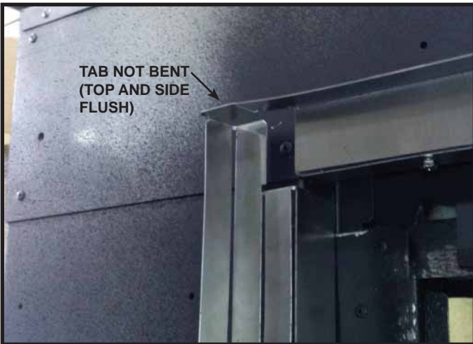
Figure 13.5 Finishing Template Bend - Operable Doors
